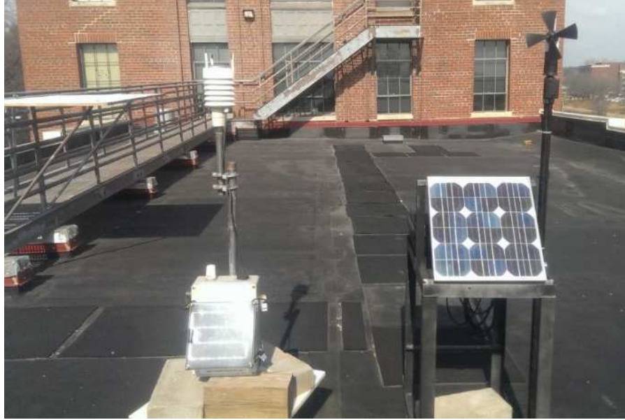
Figure 4.11 Setting of the Vaisala & Youngs anemometers on the roof of IIHR building
